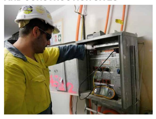
The ETU requires that all switchboards on building and construction sites (including site amenities), have a locked cover over the RCDs and circuit breaker.
